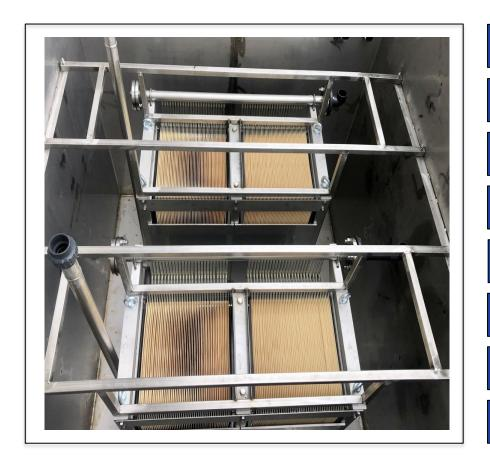
**PRODUCT** E-BOX 02-70 N. MODULES 2 (Total 140 m<sup>2</sup>) FLOW RATE 1,3 m<sup>3</sup>/h WASTE WATER **INDUSTRIAL** WATER USE **DRAIN IN SEWAGE** OEM **Confidential (Italy) END USER Confidential (Italy)** SECTOR **FOOD**
