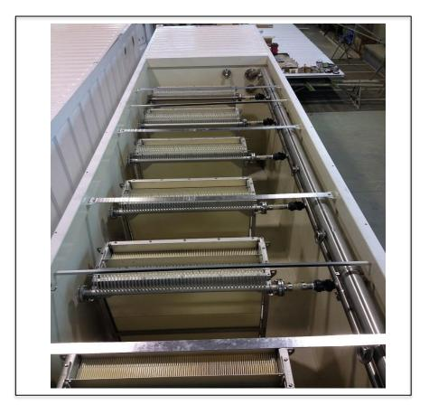
**PRODUCT** TMR140-100S N. MODULES 20 (Total 2.800 m<sup>2</sup>) 42 m<sup>3</sup>/h **FLOW RATE** WASTE WATER **MUNICIPAL** WATER USE **IRRIGATION** OEM **Confidential (Italy) END USER Confidential (Duch Antilles) SECTOR HOTEL & RESORTS**
