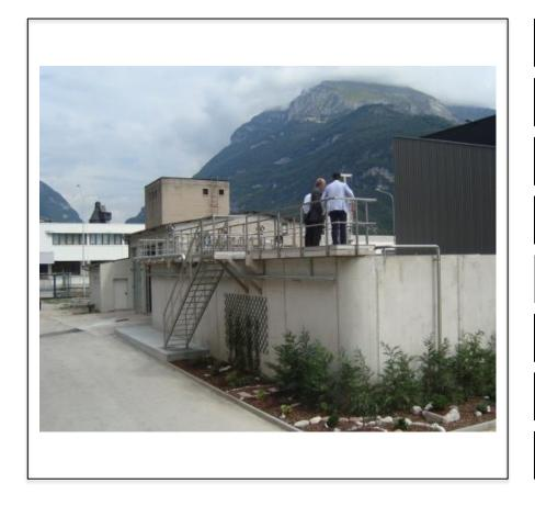
**PRODUCT** TMR140-100S 4 (Total 560 m<sup>2</sup>) N. MODULES 12 m<sup>3</sup>/h FLOW RATE WASTE WATER INDUSTRIAL LAUNDRY WATER USE **DRAIN IN SEWAGE WATER** OEM **Confidential (Italy) END USER Confidential (Italy) SECTOR INDUSTRIAL**
