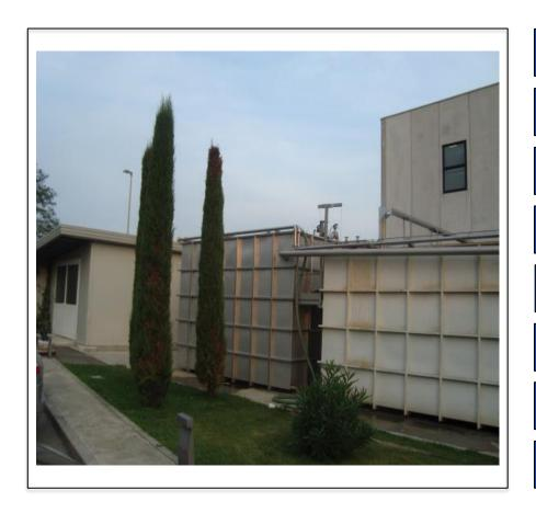
**PRODUCT** TMR140-100S N. MODULES 4 (Total 560 m<sup>2</sup>) 5 m<sup>3</sup>/h FLOW RATE WASTE WATER **INDUSTRIAL** WATER USE **DRAIN IN SEWAGE WATER** OEM **Confidential (Italy) END USER Confidential (Italy)**
