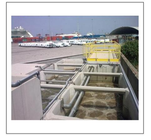
**PRODUCT** TMR140-100S 2 (Total 280 m<sup>2</sup>) N. MODULES  $4 \text{ m}^3/\text{h}$ **FLOW RATE** WASTE WATER **INDUSTRIAL** WATER USE **SEWAGE DISCHARGE** OEM **Confidential (Italy) END USER Confidential (Italy) SECTOR CRUISE SHIPS**
