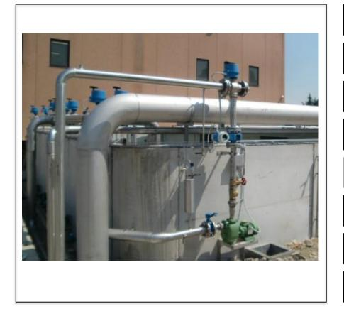
**PRODUCT** TMR140-200W N. MODULES 4 (Total 1.120 m<sup>2</sup>) 20 m<sup>3</sup>/h **FLOW RATE** WASTE WATER **GRAPE PROCESSING** WATER USE **SEWAGE DISCHARGE** OEM **Confidential (Italy) END USER Confidential (Italy) SECTOR WINERY**
