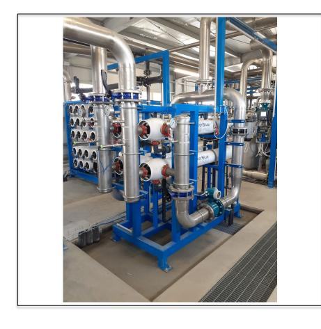
**PRODUCT FILTERBLUE-BL-03 FLOW RATE** 216 m<sup>3</sup>/h (4 x 54 m<sup>3</sup>/h) WATER **RO PRETREATMENT APPLICATION BRACKISH WATER** WATER USE **INDUSTRIAL WATER** OEM **Confidential (Italy) END USER Confidential (Italy) SECTOR FOOD**
