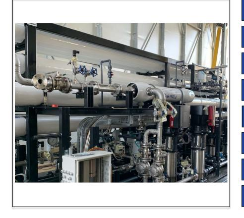
**PRODUCT FILTERBLUE-BL-02** FLOW RATE 36 m<sup>3</sup>/h WATER **BRACKISH APPLICATION RO PRETREATMENT** WATER USE **PROCESS WATER** OEM **Confidential (Italy) END USER Confidential (Italy) SECTOR INDUSTRIAL**
