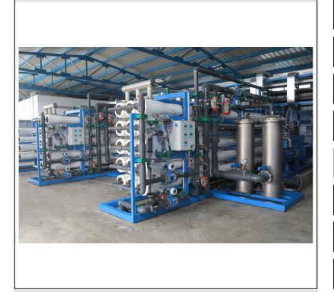
**FILTRO FMG-22 PRODUCT Cartridges N95F FLOW RATE** 4 x 88 m<sup>3</sup>/h WATER **BRACKISH WATER APPLICATION RO PRETREATMENT** WATER USE **DRINKING WATER** OEM **Confidential (Palestine) END USER Confidential (Palestine) SECTOR**
