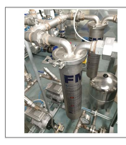
FILTRO FM-0 **PRODUCT Cartridges N95F** 2 X 10 m<sup>3</sup>/h **FLOW RATE** WATER **BRACKISH WATER APPLICATION INDUSTRIAL** WATER USE WATER FOR SOFT DRINKS OEM **Confidential (Italy) END USER Confidential (Italy) SECTOR BEVERAGE**
