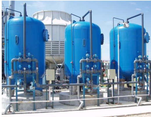
Photo of Reverse Osmosis pre-treatment with sand filters
