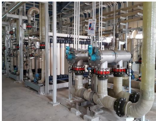
Photo of a reverse osmosis pre-treatment with self-cleaning filters and ultrafiltration modules
