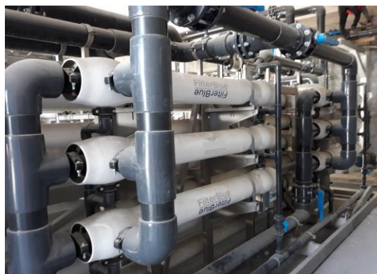
Photo of Reverse Osmosis pre-treatment with cartridge filter housings
